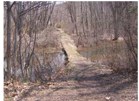
Bridge over canal
