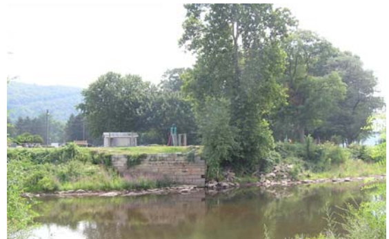
Retaining wall in location of former Water House
